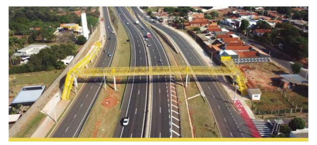
The widening of 19 kilometers of the Comandante João Ribeiro de Barros Highway (SP-294), between Marília and Oriente, has been completed and is now open to drivers. The twinning works along this section included additional pedestrian overpasses and the construction or upgrading of four onramps and turnarounds. SP-294 serves as a vital transportation artery, stretching from Bauru across the state to Panorama, near the border of Mato Grosso do Sul, with links to other major highways.
